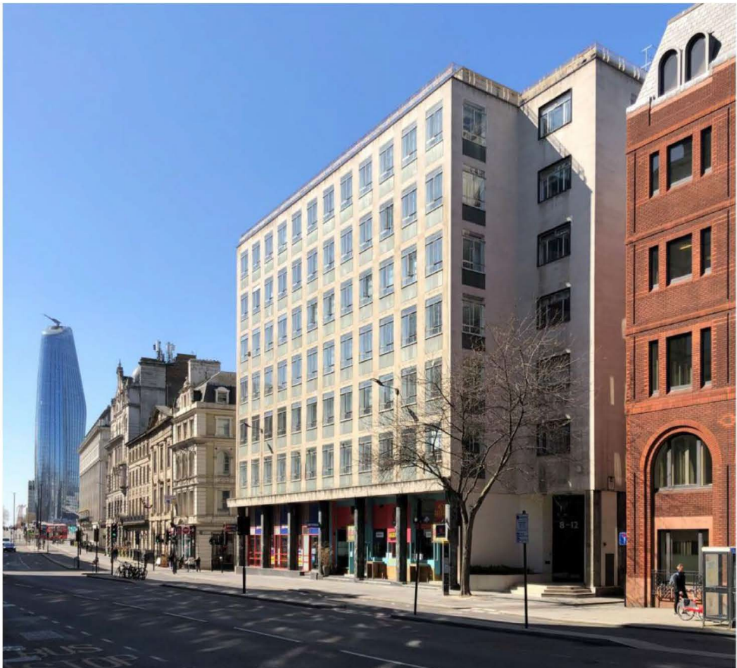
2. View from New Bridge Street looking south
